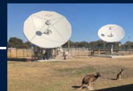
ROC at Telstra Landing Facility
